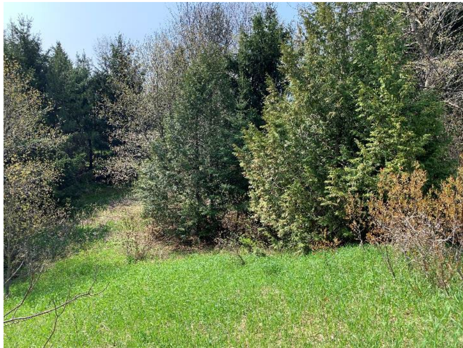
Photograph 12: Alternative view of slope with grass vegetation, from top of bank
