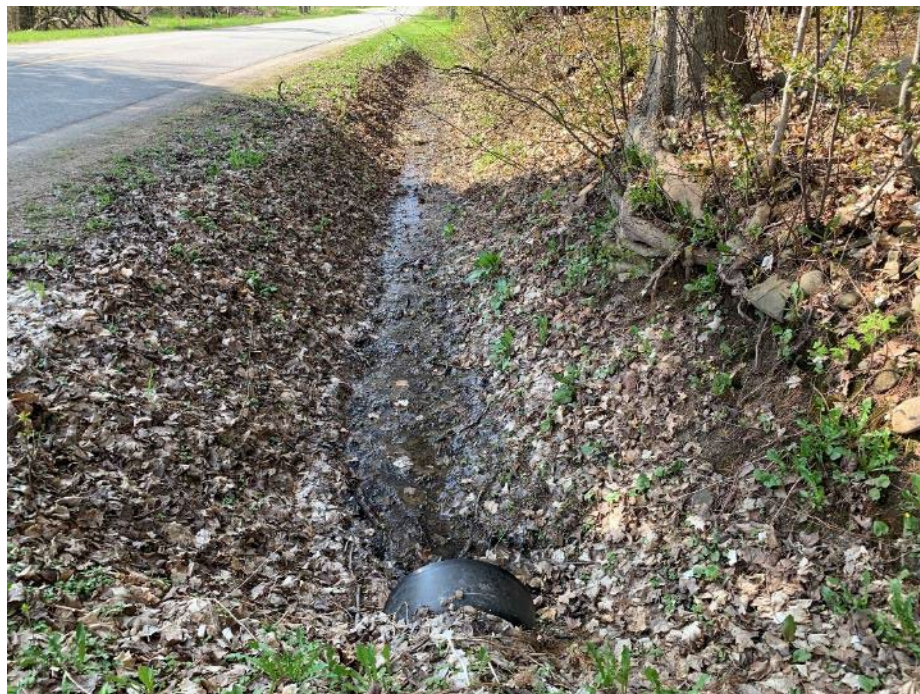
Photograph 7: View of ditch area and Main Street, looking south
