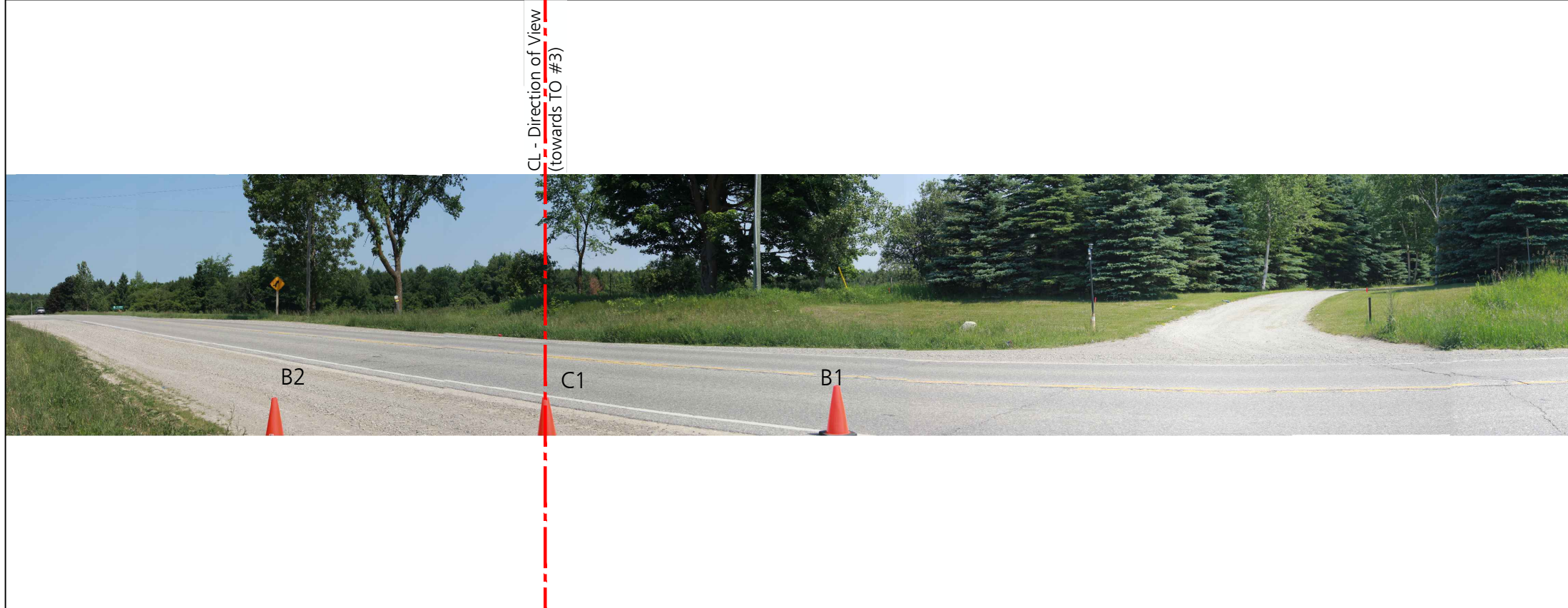
Existing Conditions Photograph (On Leaf Conditions - June 21, 2023)
