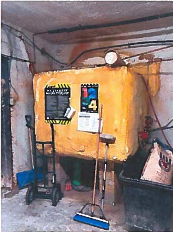
Figure 22: Zamboni Hot Water Storage Tank
