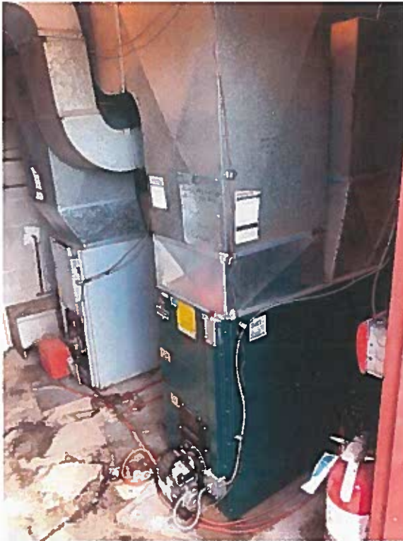
Figure 18: Common Area Oil Furnaces
