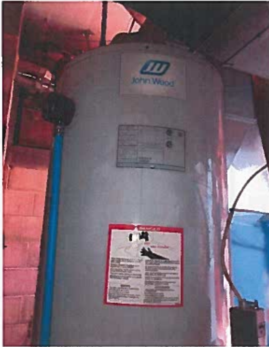
Figure 21: Domestic Hot Water Tank
