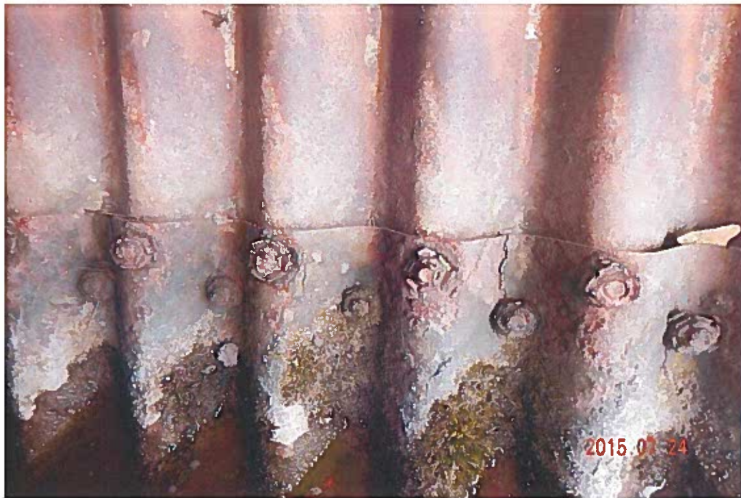
Photo 4: Internal Defects – Severe Corrosion of Bolts
