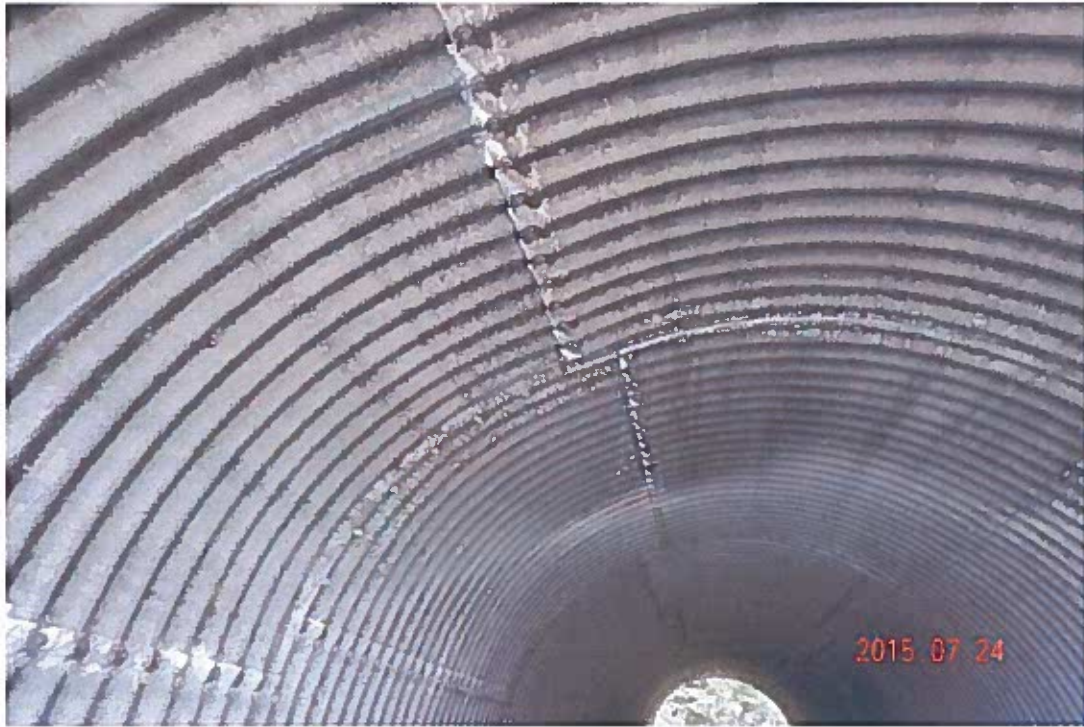
Photo 7: Internal Defects – Water Penetration
