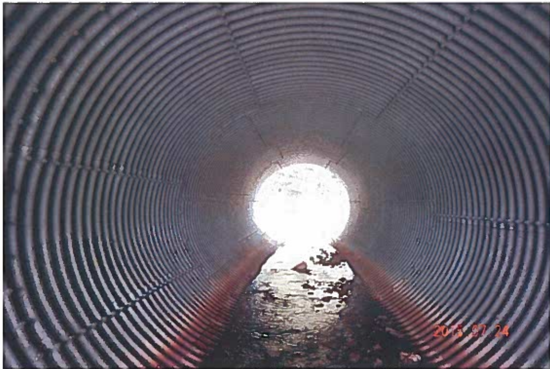
Photo 8: Internal Defects – Severe Corrosion of Culvert Floor
