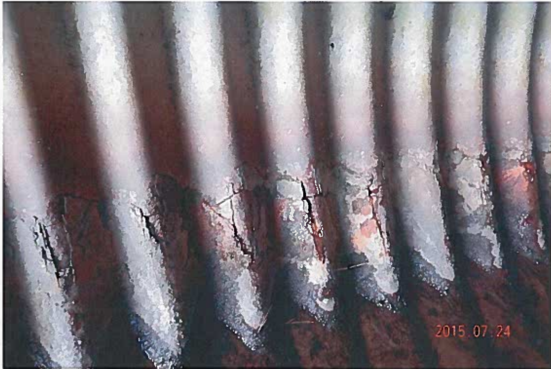
Photo 5: Internal Defects – Severe Section Loss
